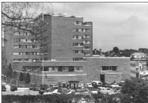
By 1977, the two aboveground stories depicted in the foreground of this photo had been added to the Cancer Center.
