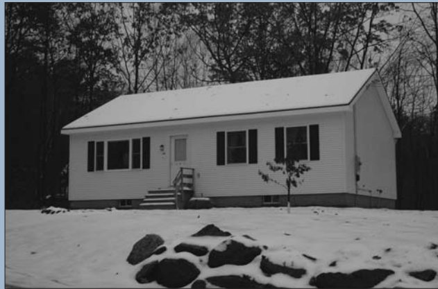
The foundation for this cozy home, a Habitat for Humanity project, was excavated by the construction firm that's handling DHMC's expansion.
